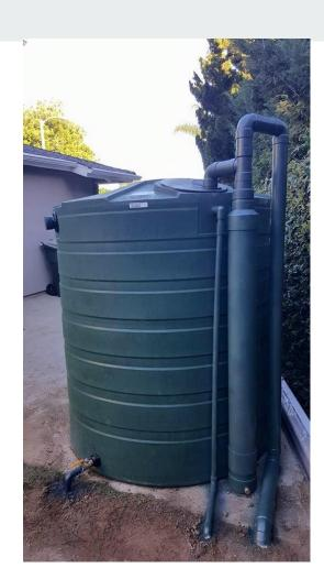
Small/Medium sized system: 865 Gallons. Polyethylene construction. Dimensions 5'1" diameter, 6'3" height.
